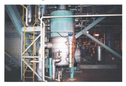
The concentration of undesirable solid particles in boiler water can be reduced by means of a continuous cleaning or draining system. The blowdown tank receives continuous discharge from the boiler drum and the discharge from the vapor generator at various temperatures and pressures. The waste tank can also be used as an automatic drainage system for the vapor generator when the generator is being drained for maintenance.
