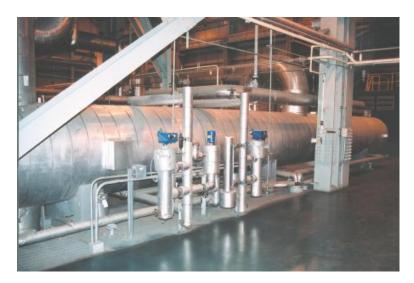
The feed water heater raises the temperature of boiler water by drawing vapor from the turbine. The water first enters a low pressure heater to heat it, then enters a deaerator to remove excess oxygen, and then enters a high-pressure heater to further heat and pressurization. According to the ASME standard, each heater must be equipped with two independent liquid level control loops.
