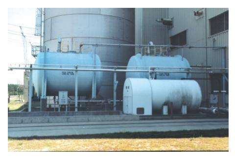
The generator and gas turbine have an integrated lubrication system to prevent damage caused by excessive friction. A part of lubricating oil is usually used in the hydraulic oil system. Lubricating oil is usually stored in integrated stainless steel and carbon steel tanks with level monitoring.
