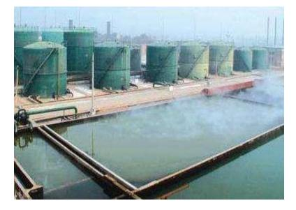
Oil field sewage mainly includes crude oil effluent (also known as oil production), drilling sewage and other types of oily sewage in the station. There are many ways to treat oilfield sewage according to the factors of oilfield production and environment. When the oil field needs water injection, the oil field sewage is treated and injected back into the formation, and the suspended matter and oil in the water should be strictly controlled at this time to prevent the damage to the formation.
