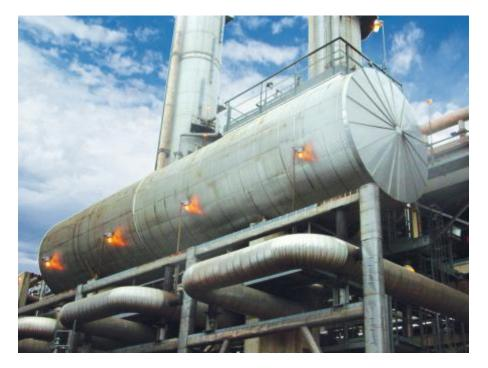
In the preheating system of the distillation tower, a pre-flash tank system separates the steam generated before preheating from the heater or main distillation tower. This can prevent the heater from overheating combustion or pressure drop and reduce the steam load of the distillation tower to avoid flooding.
